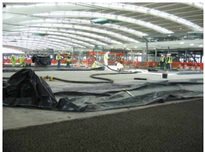
Figure 2: Heathrow Terminal 5 has chosen to use lightweight aggregate.
