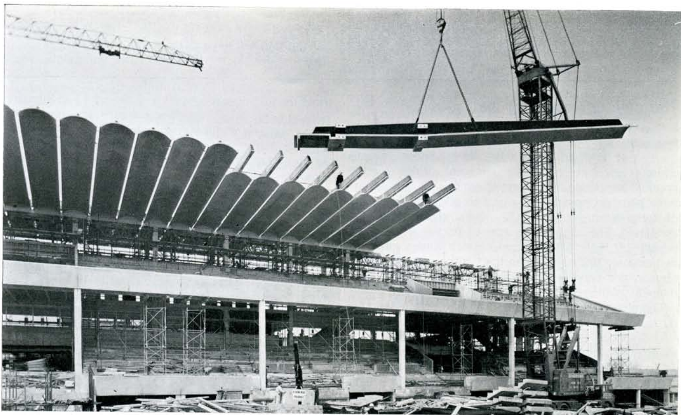
Figure 5 Erecting a roof unit.
