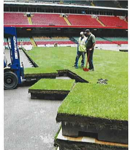
Secondary aggregate is used as a efficient drainage medium in some high profile venues.
